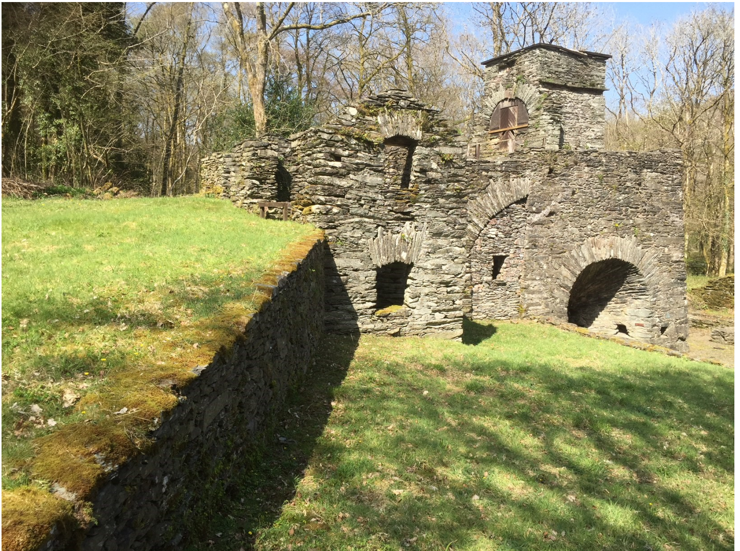
Duddon Furnace. Note the vaulted masonry arch of the casting arch on the right of the picture. This is unlike the bressemer-beam construction often pictured in textbooks.
